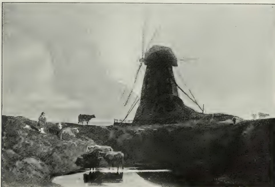
DRAINING MILL, LINCOLNSHIRE.
